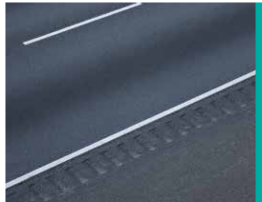
Figure 2. Shoulder rumble strip on Interstate 95 (North), Stafford County, Va. (Image: James Scott Baron, ATSSA)
