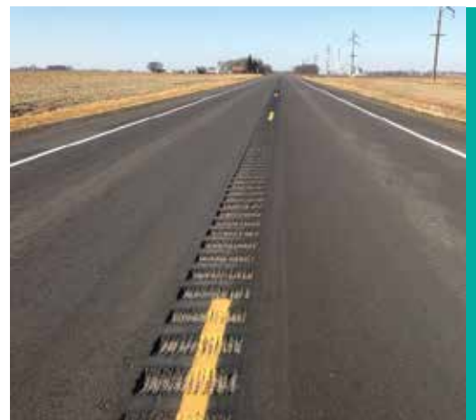
Figure 3. A sample of milled centerline rumble strips (Image: Neal Hawkins, Center for Transportation Research)
