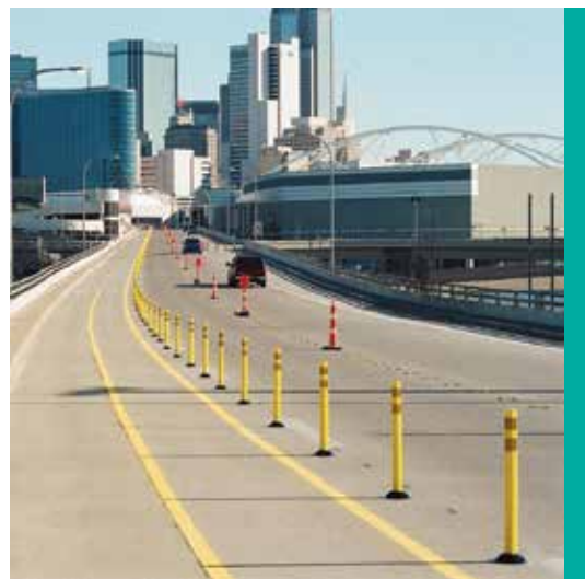
Figure 23. Flexible channelizing devices (Image: Pexco LLC)
