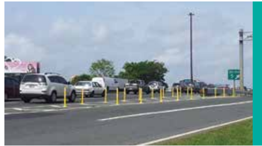
Figure 22. Flexible channelizing devices (Image: Pexco LLC)
