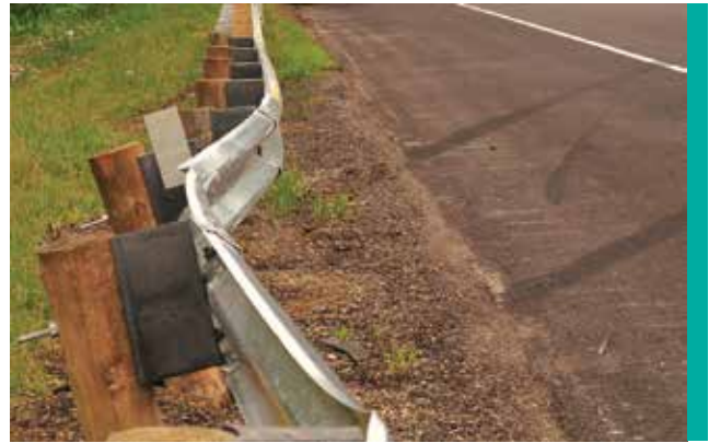
Figure 33. Note the skid marks of the vehicle that struck this guardrail. Crashes such as this are often unreported, especially if the vehicle operator can drive away. A dedicated, stable source of federal funding is important to ensure that these life-saving safety devices are repaired in a timely manner (Image: Karen Boodlal, KLS Engineering)
