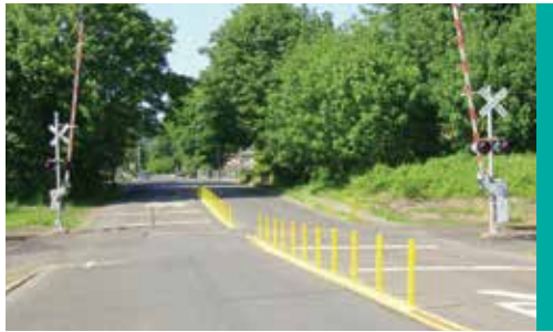
Figure 21. Flexible channelizing posts at a railroad crossing, Washougal, Wash. (Image: Pexco LLC)
