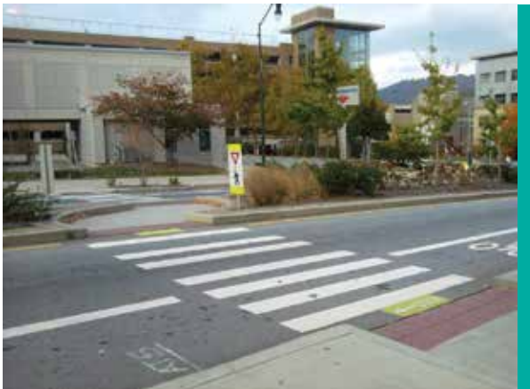
Figure 25. An Asheville, N.C., mid-block pedestrian crossing with a pedestrian refuge island (Image: Lyubov Zuyeva)
