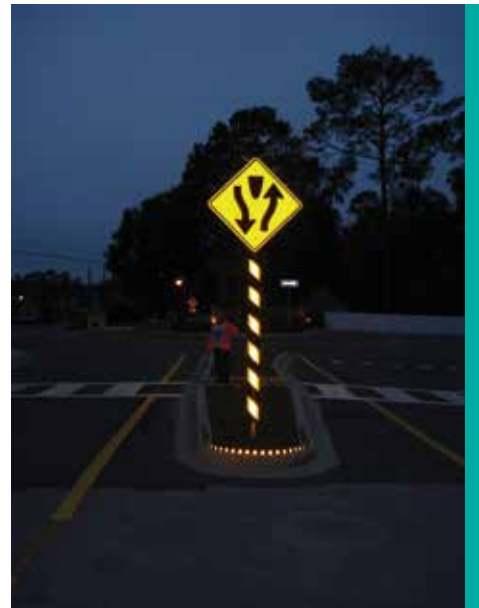
Figure 26. Reflective material on the concrete curb below the sign and its post alerts motorists there is a curb on the roadway (Image: Professional Pavement Products)
