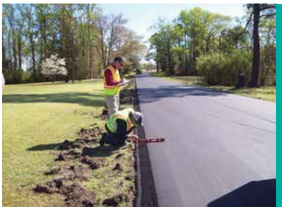
Figure 19. Federal Highway Administration's (FHWA's) Andy Mergenmeier and Chris Wagner gathering data on a new Safety Edge SM project (Image: Frank Julian, FHWA)
