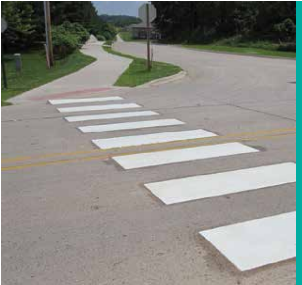
Figure 10. A highly visible, clearly marked pedestrian crosswalk (Image: Neal Hawkins, Center for Transportation Research)
